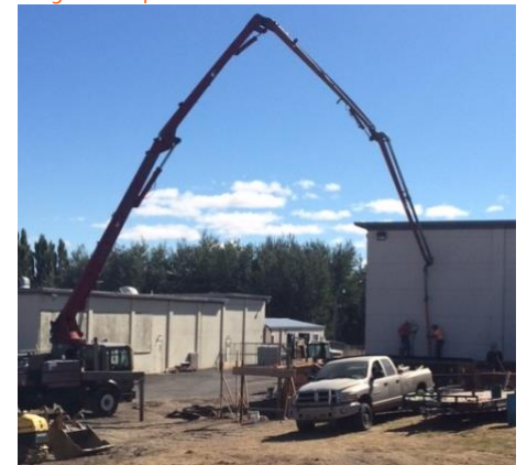
Kitchen Building – Photo taken September 21, 2015
