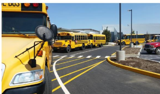
New bus lane approach and drop off/pickup zone.
