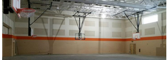
Above: The gym basketball hoops are in and the floor will be poured soon.
