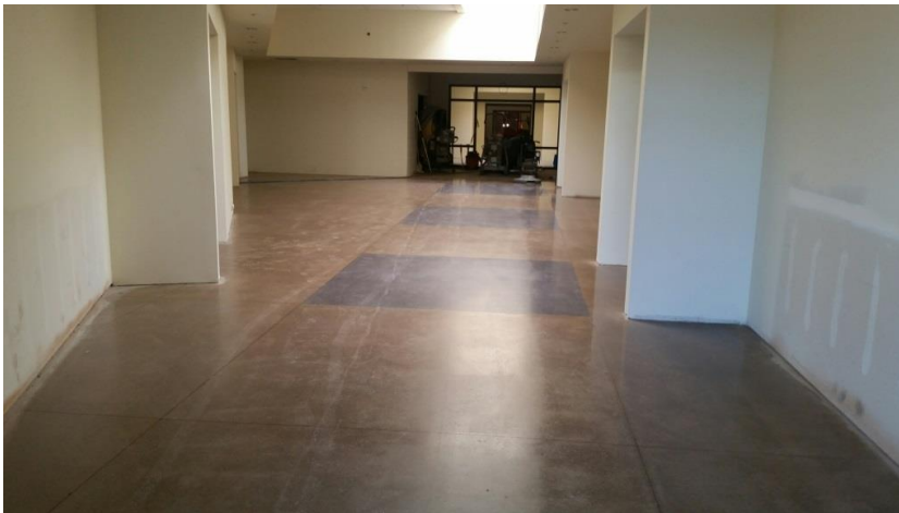
Above: The polished concrete outside the Pre-K through 3 rd grade classrooms.
