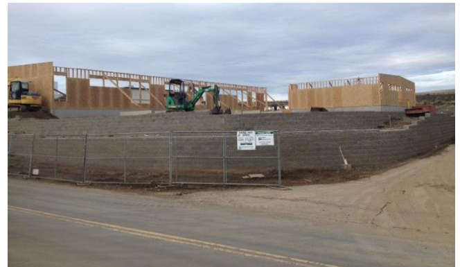
Above: Exterior walls are being framed, sheathed, stood and braced.
