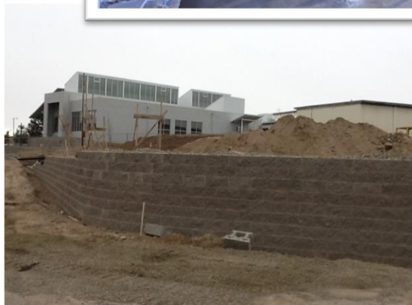
Above: Retaining wall at north side
